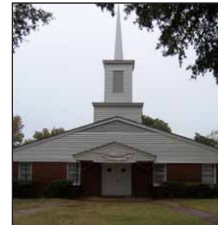
Below: Chief Corner Stone recently purchased and began meeting in the buildings of the former Northview Baptist Church in Frayser.
